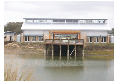
East Metro Community Pavilion at 18667 Blake Manor Road
